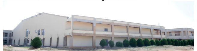
Expansion of modular theatre (70% completed)
