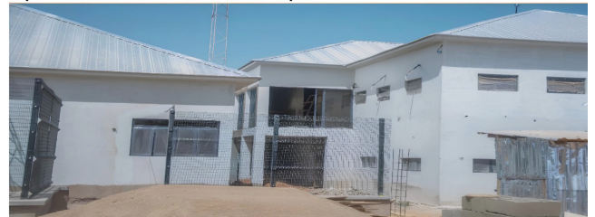
Construction of the tuberculosis reference laboratory JUTH
