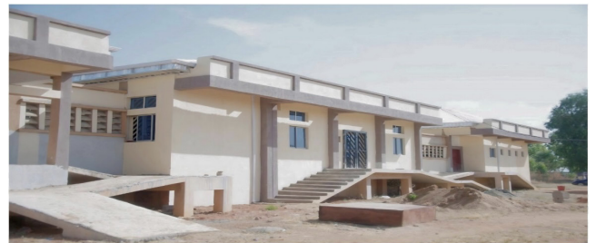
Construction of psychiatry complex phase 2
