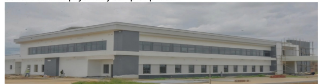
Construction of NSIA/JUTH Advanced Diagnostic Center
